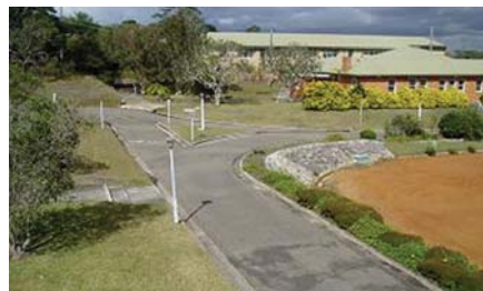
On road - Utilising existing low traffic roads, North Head, Manly
